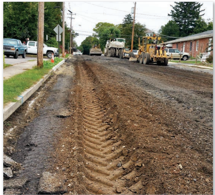
Full Depth Reclamation on Pennsylvania Ave (2015)
