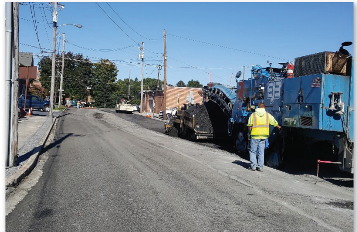
Cold In-Place Recycling on Eighth Street (2016)
