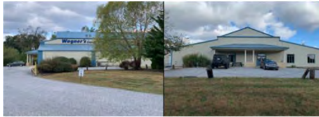
Old Wagner Supply Building – Now Only Used for Storage
