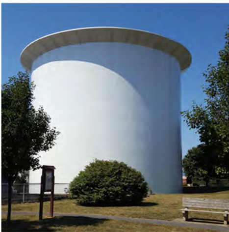
Birkinbine Tank Last Re-Painted in October 2015
