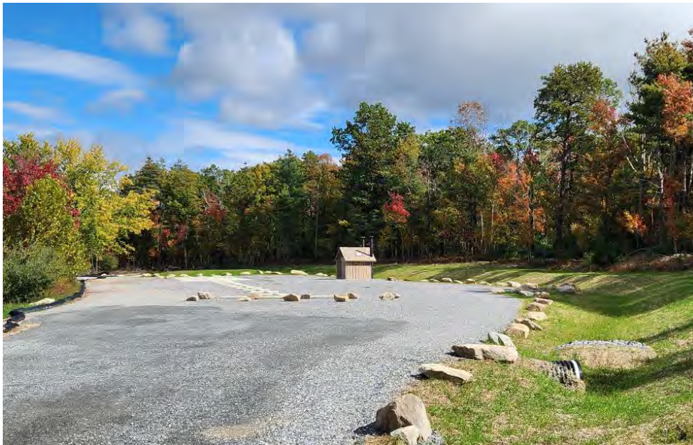
Newly Constructed Long Pine Parking Area – Fall 2023
