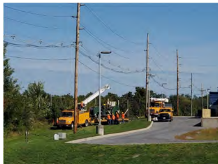
Line Crews Installing Underground Cable and Overhead Messenger for Fiber Network
