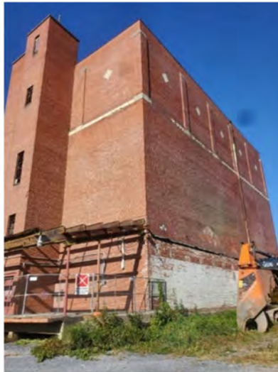
Old Cold Storage Building before Demolition
