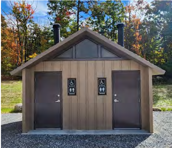
Long Pine CXT Restroom – Fall 2023
