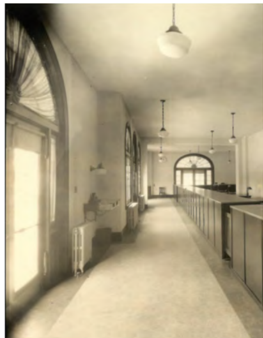
The original front counter in what-is-today, the Admin. Office Suite
