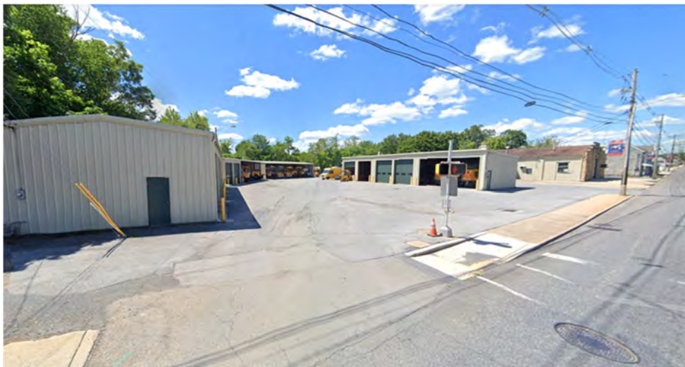
Loudon Street Public Works Facility
