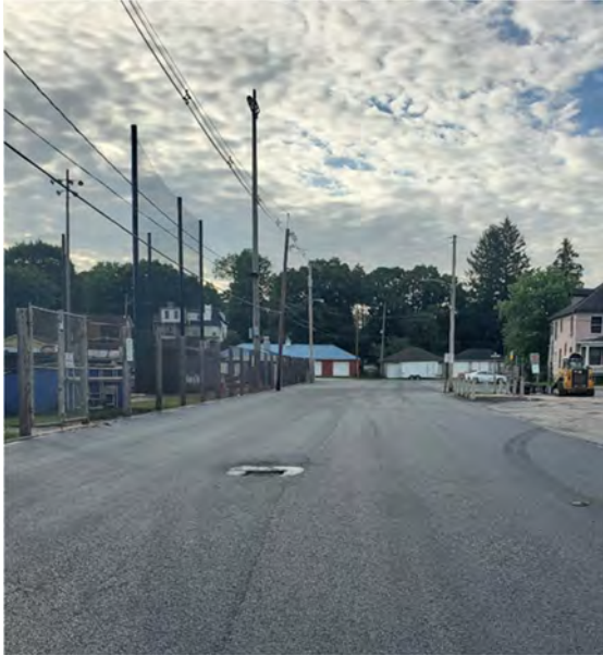
Vine Street Box Top Replacement
