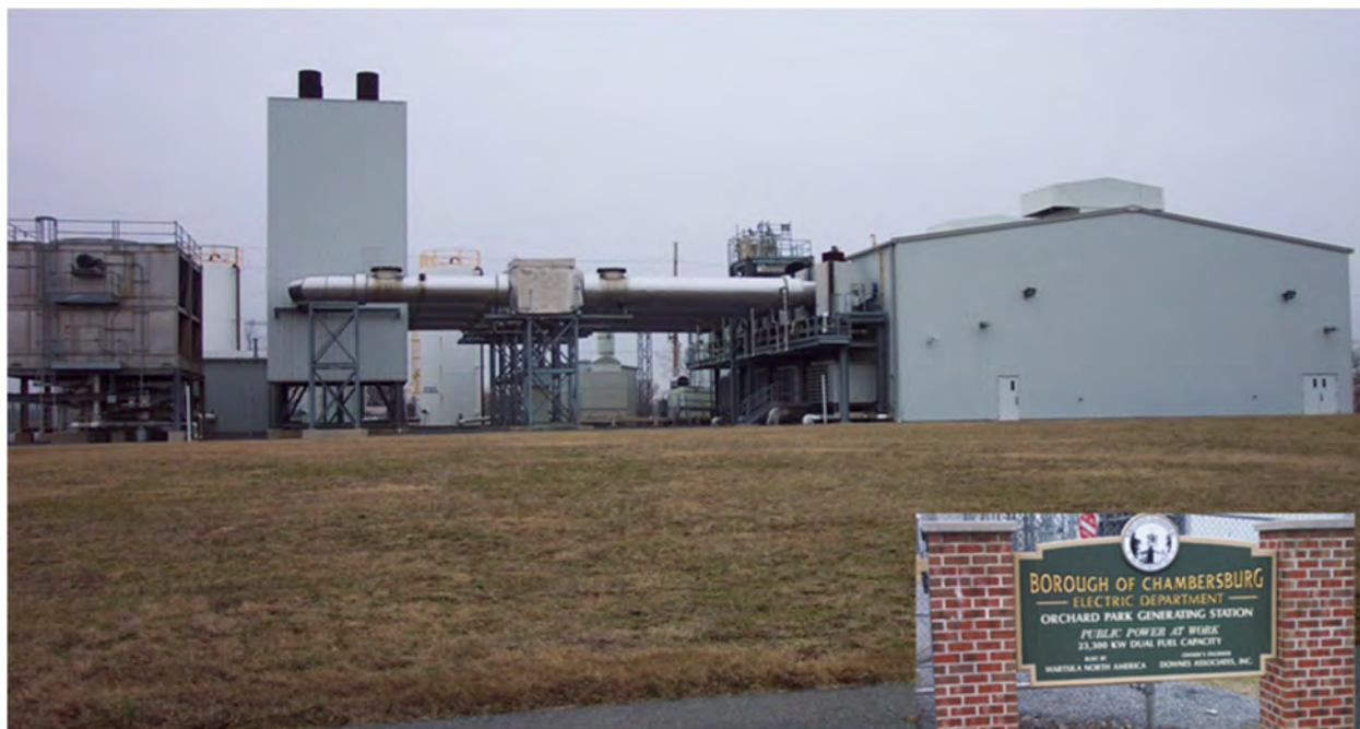
Orchard Park Generating Station (OPGS)
