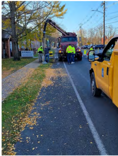
Digging a pit for the new guiderail along Fifth Avenue
