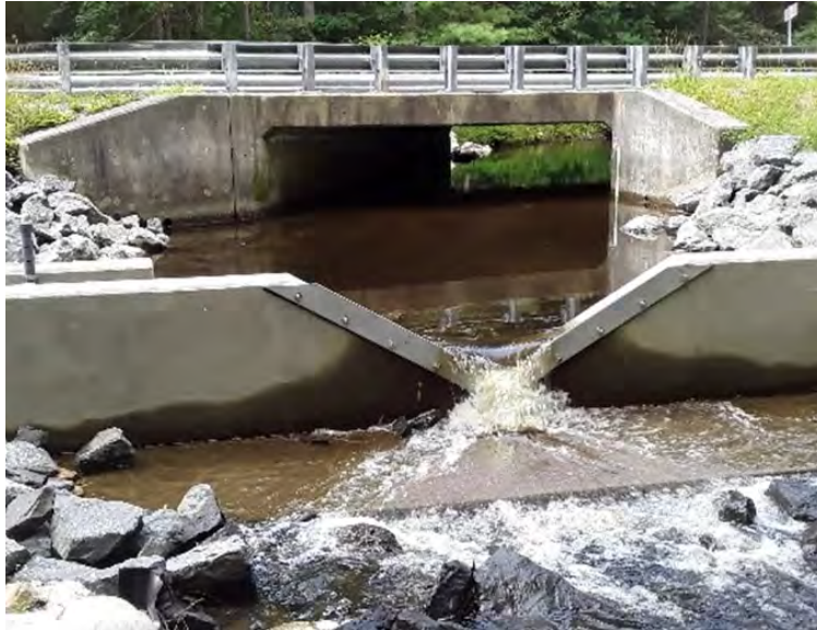
Conococheague Weir in Operation
