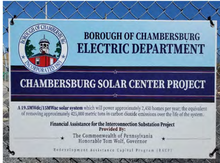
Interconnection Substation Sign
