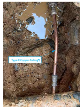
Water Service After Gooseneck Removal
