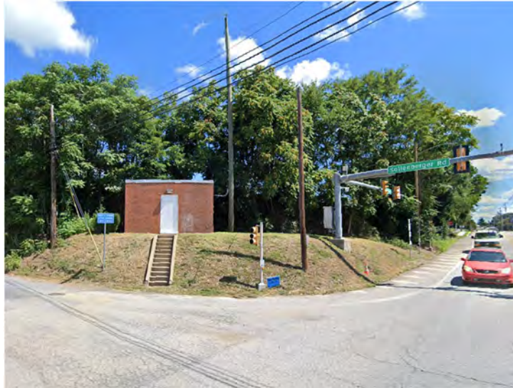
The Interconnection Pump Station at Sollenberger Road between the Chambersburg Water System and the Bear Valley Joint Intermunicipal Authority
