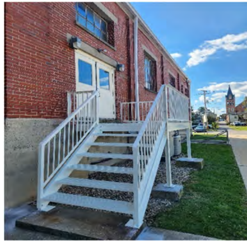
Replaced exit Staircase off Gym 1 side entrance. Intended to sandblast and powder coat it, but they were too corroded and ultimately needed to be replaced. These are aluminum, powder coated, with open treads that should not rust.
