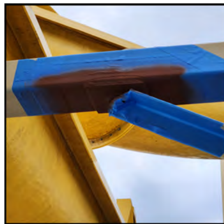
Aquatic Center slide repairs
