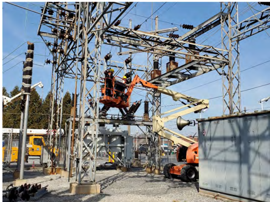
Investment in Infrastructure because of the 2019 Bond Issue
