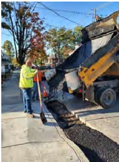
Borough Employees Fixing Street After Curb Replacement
