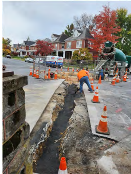
Glen Street Fountain Restoration Progress
