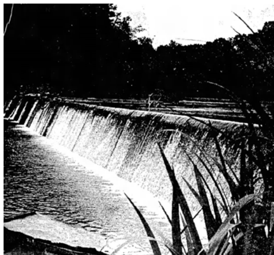
The Second Siloam Dam
