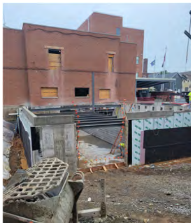
Addition to the Police Station under construction
