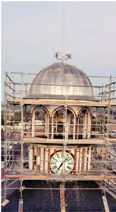
Clock Tower being restored in 2022
