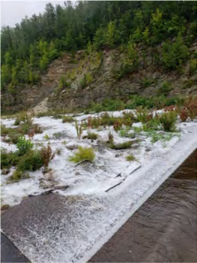
Long Pine Spillway – July 2018
