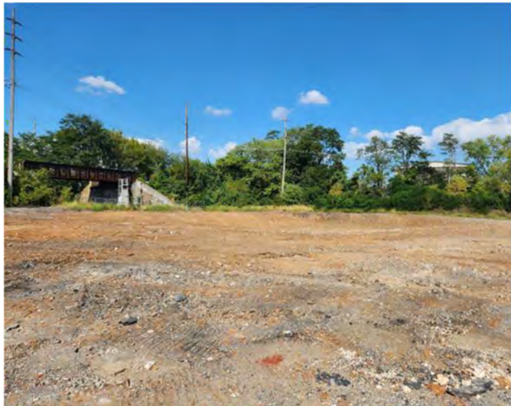
Site of former Cold Storage building after demolition
