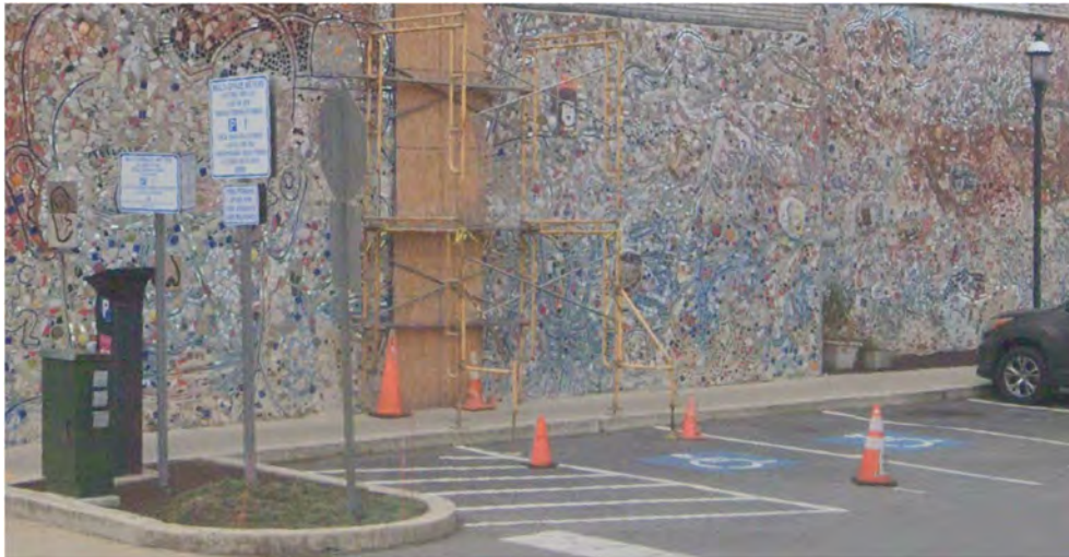
One of two existing parking kiosks in the Rosedale Parking Lot
