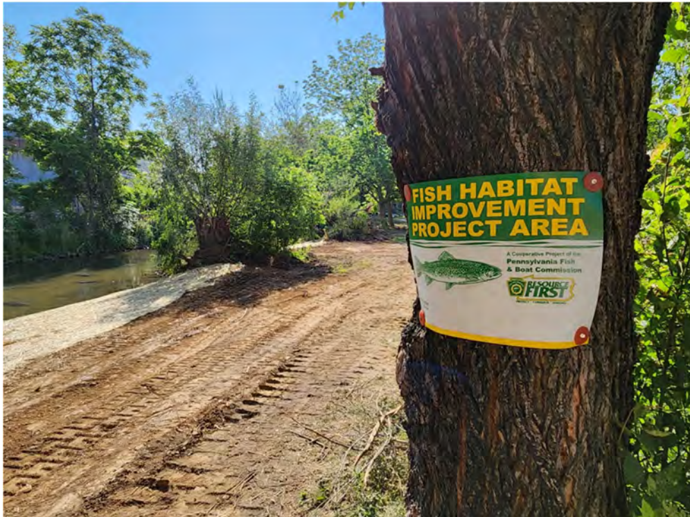
Falling Spring Streambank Restoration Project
