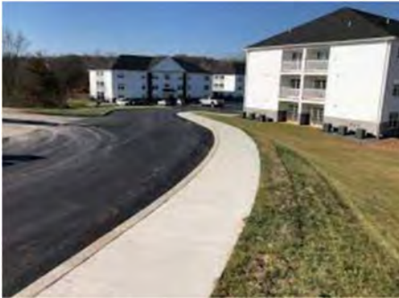
Creekside Apartments, Hollywell Ave.
