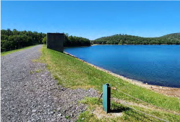
Long Pine Run Dam Control Tower and Access Road
