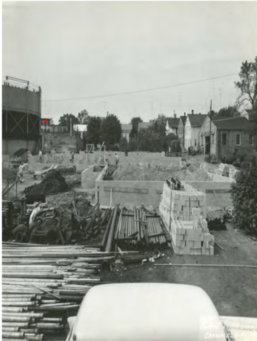
Service Center under Construction, with MGP Tank Top Left
