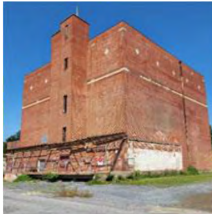
Cold Storage building prior to demolition
