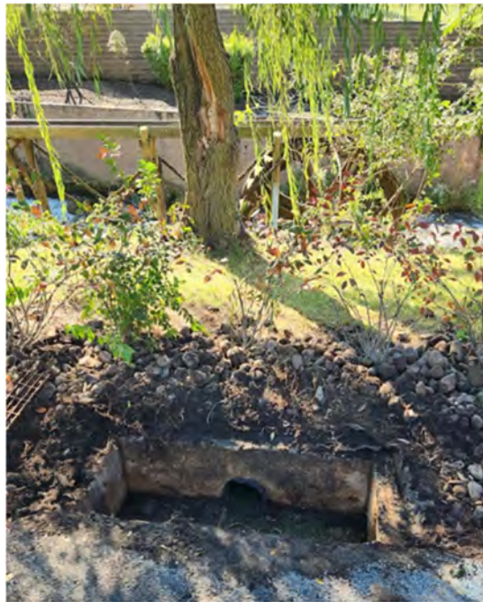
Storm Water Inlet at the Water Wheel, Chambers Fort Park
