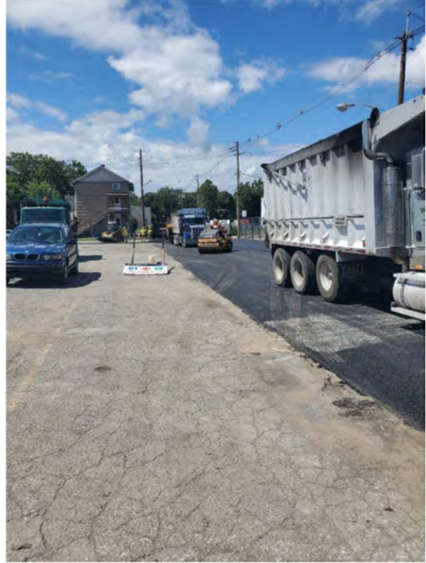
Paving Operation – Vine Street
