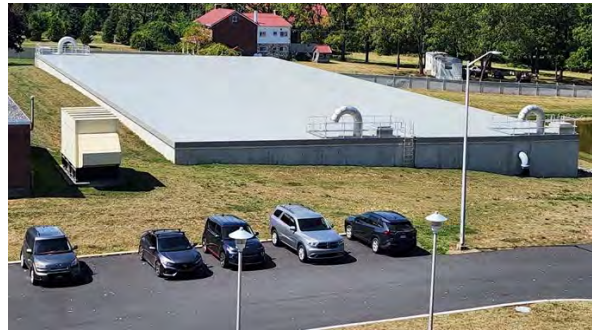
WTP Clearwell 2 – 2.5 MG
