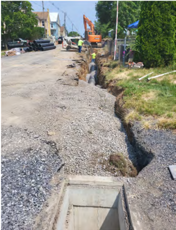
Center Street Storm Sewer System Improvements
