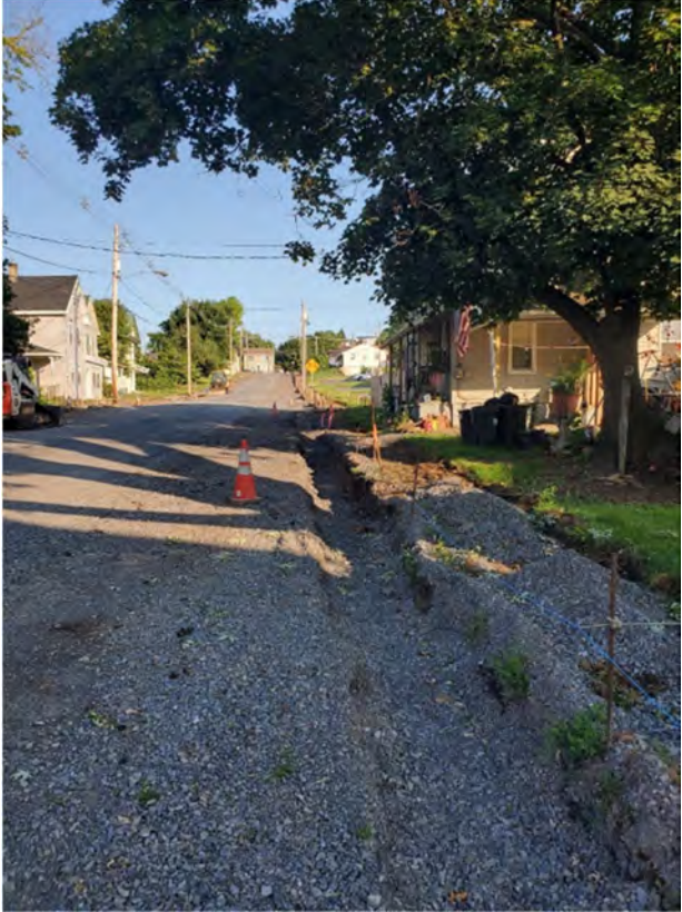
Center Street – Curb and Sidewalk Replacement
