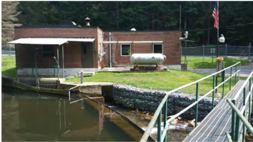
The Original Water Intake in Caledonia Still in Use
