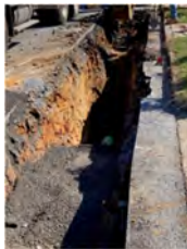
Sewer Main Installation
