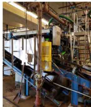
Aging Equipment – Belt Press
