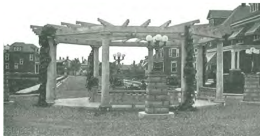
Original Glen Street Fountain and Pergola (gravel streets)
