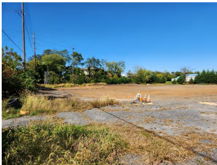
Former Cold Storage site after demolition
