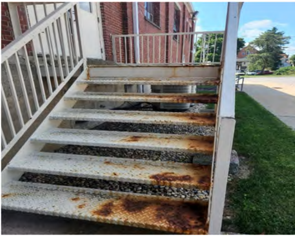
Replaced exit Staircase off Gym 1 side entrance. Intended to sandblast and powder coat it, but they were too corroded and ultimately needed to be replaced. These are aluminum, powder coated, with open treads that should not rust.
