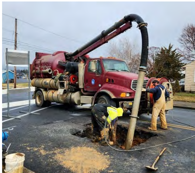
Water Service Excavation with Vac Truck
