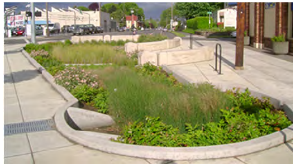
Out-of-Town Example of Stormwater Best Management Practice (BMP) on Private Property
