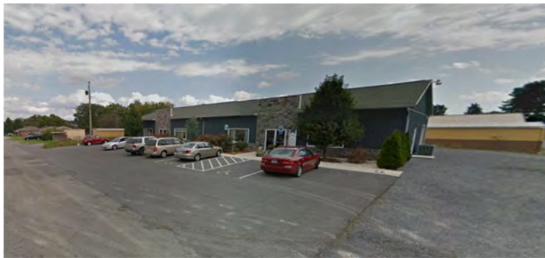
Office Building Occupied at 1332 S. Fourth Street
