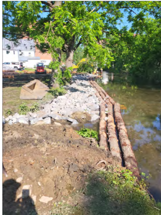
Falling Spring Streambank Restoration Project
