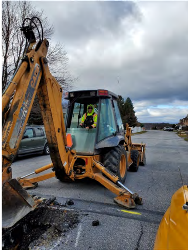
Digging a test pit in Laurich Meadows to test pavement conditions
