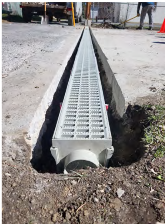
Liberty Street Storm Sewer System Improvements
