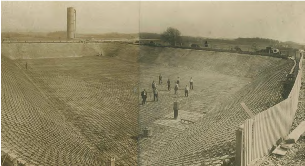
Dull Hill Reservoir in Guilford under Construction
