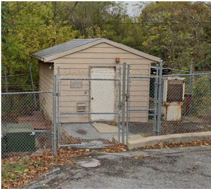
Laurich Meadows Pump Station
