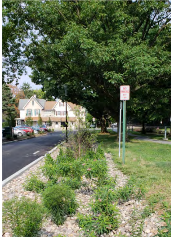
Rhodes Drive Stormwater Management Facility BMP Maintained by Storm Sewer Utility
