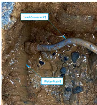
Water Service Before Gooseneck Removal
