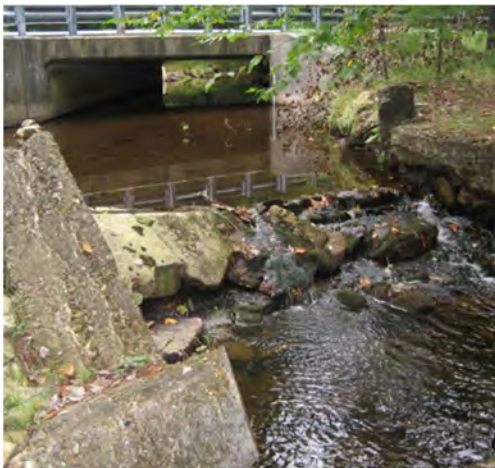
Conococheague Weir Condition
