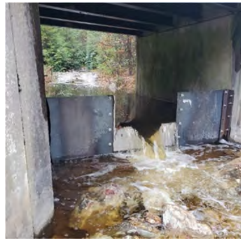
Long Pine Run Weir
