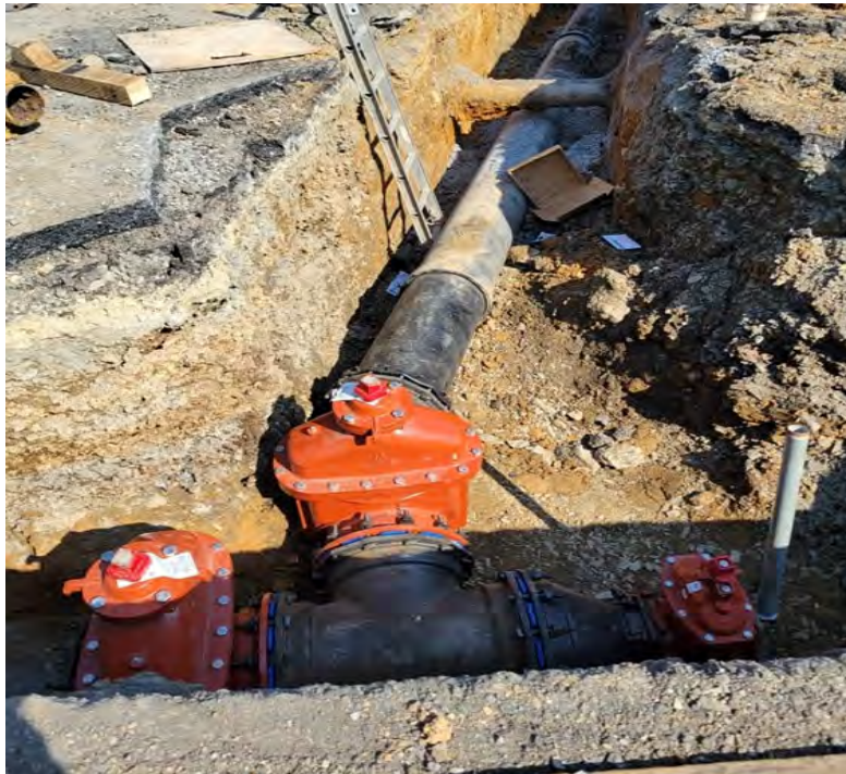
Chambers Street/Reservoir Hill Water Main Extension Project Valve Installation
